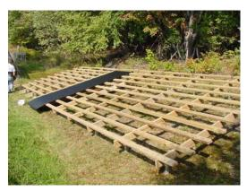
Photo to the left shows the completed rack with all decking in place. Panels are now fastened to the decking in the same manner as on a conventional roof.
