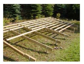
After all the rafters are bolted to the posts the decking  $2 \times 4$ 's can be fastened to the rafters. The spacing for the decking is approximately 13 to 14 inches on center depending upon panel length. The overall spacing on the top and bottom planks are one inch less than the panel length.
